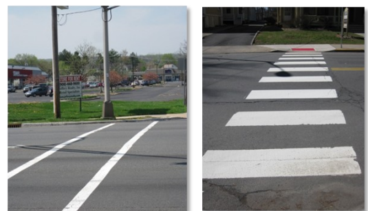
A standard crosswalk pattern (left) and a continental pattern (right)
