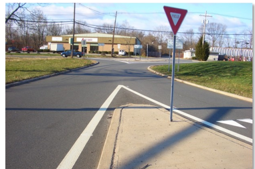
The merge of South Main Street (left) and traffic exiting Route 202 (right) is uncomfortable for cyclists
