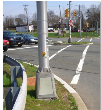
The existing crosswalk at Voorhees Corner Road & Route 202 doesn't have sufficient standing space or any curb ramps
